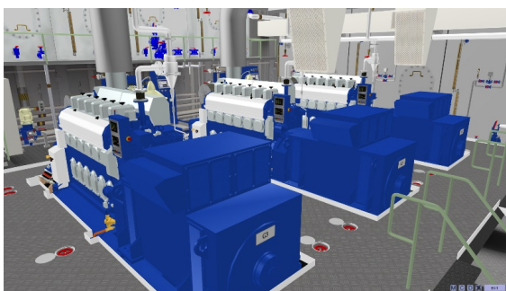
Figure 4. Auxiliary Diesel Generators
