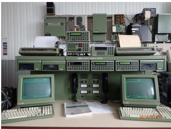
Picture 3. GMDSS console TGS-2000 (Real equipment)
