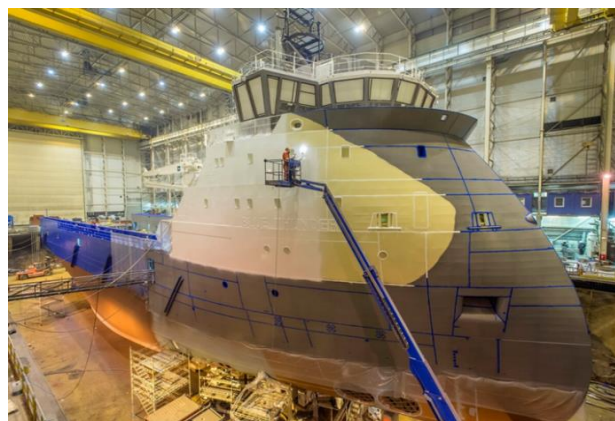
Fig. 4. Construction of the X-BOW building (Norwegian company Ulstein).
